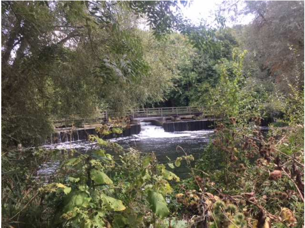
Bridge over River Avon at Downton by John Gurney
